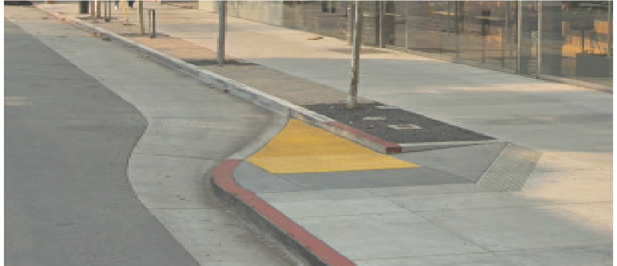
Curb ramp at bulb-out
