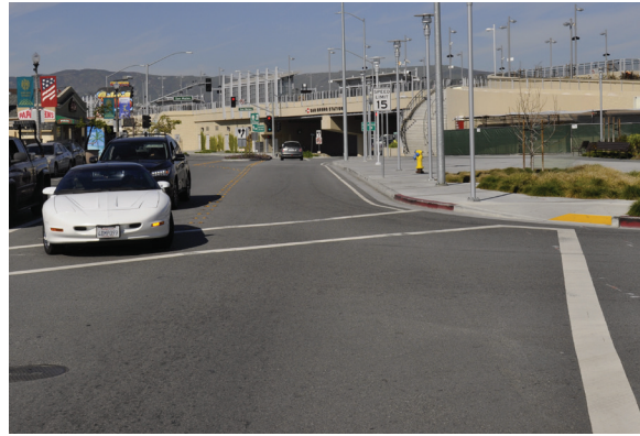
Newly replaced asphalt
