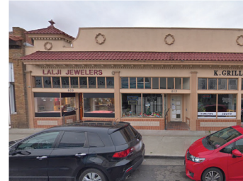
609-617 San Mateo Ave Mission Revival, 1909
