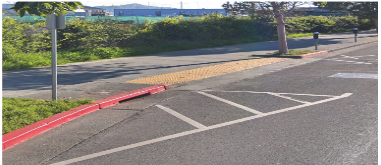
Mid-block curb ramp
