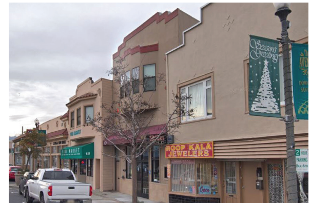
Wide Light Pole Spacing
