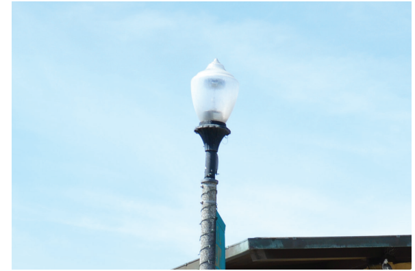
Existing Light Poles
