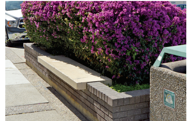
Raised planter with overgrown planting
