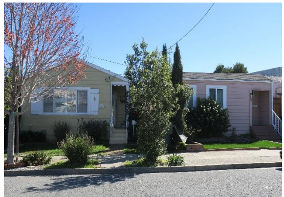
Figure 21: 283 and 289 Florida Avenue.
