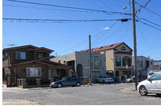
Figure 11: 349, 363, 373, and 381 Taylor Avenue. These properties look north to 324 Florida Avenue. All are contributors to the identified Cupid's Row Historic District.
