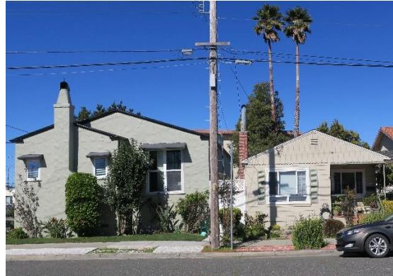
Figure 17: 202 Carlton Ave and 148 Cupid Row, both contributors to the identified Cupid's Row Historic District.
