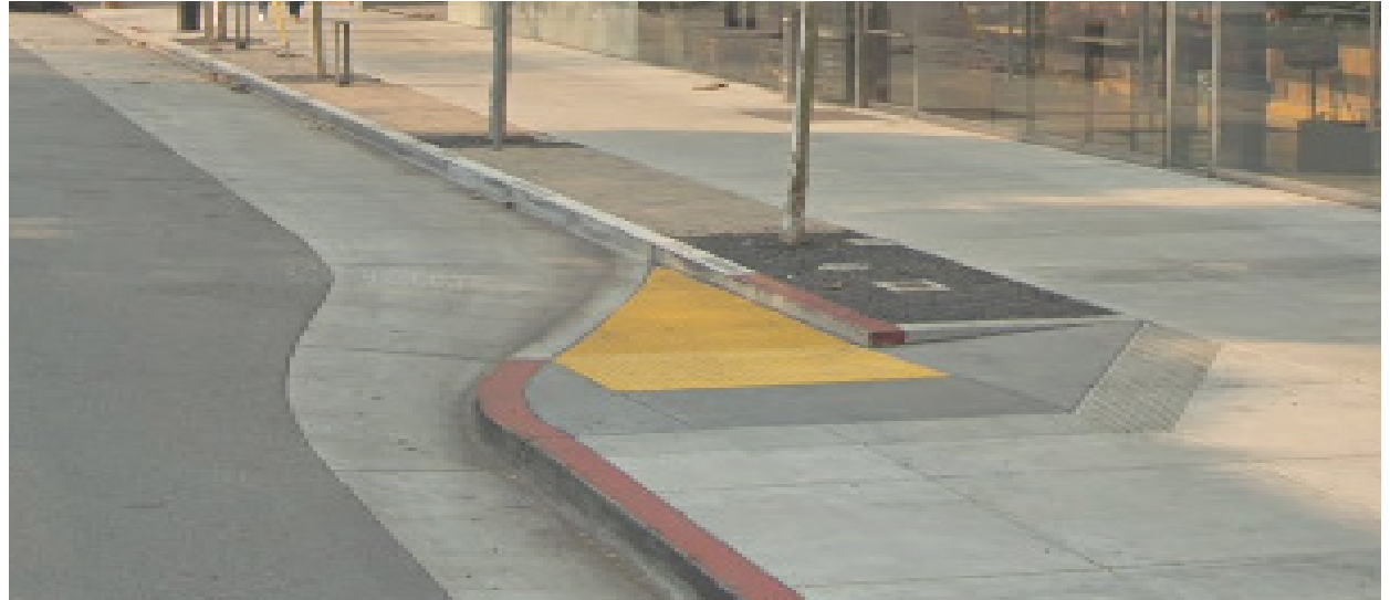
Curb ramp at bulb-out
