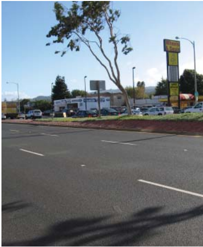
El Camino Real with a wide right-of-way dominated by vehicular traffic.
