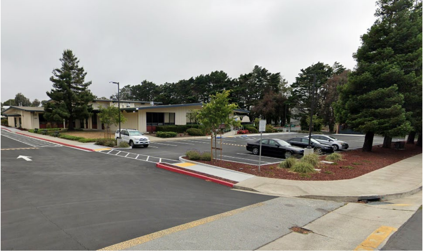
Figure 16. Recent upgrades on school grounds have improved the connection between school buildings and the crosswalk on Commodore Dr.
