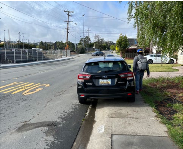
Figure 11. Rolled curbs on Millwood Dr allow vehicles to block the pedestrian path of travel.
