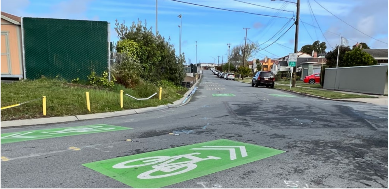
Existing green bike markings on Magnolia Ave adjacent to Capuchino High School.
