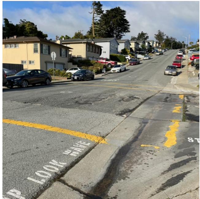
Figure 25. The existing crosswalks at Cottonwood Dr/Rollingwood Dr.
