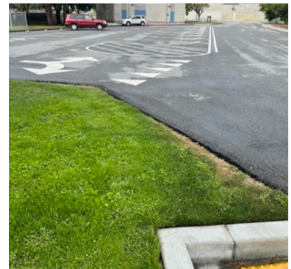
Figure 6. A dead-end sidewalk connection to the Lion's Park parking lot.
