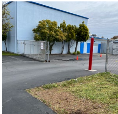
Figure 5. The southern alley entrance.
