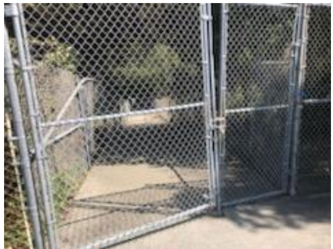
Figure 20. The locked gate to the pedestrian path.
