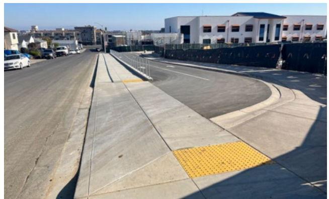
Figure 3. The newly constructed pick-up/drop-off loop on Angus Ave.
