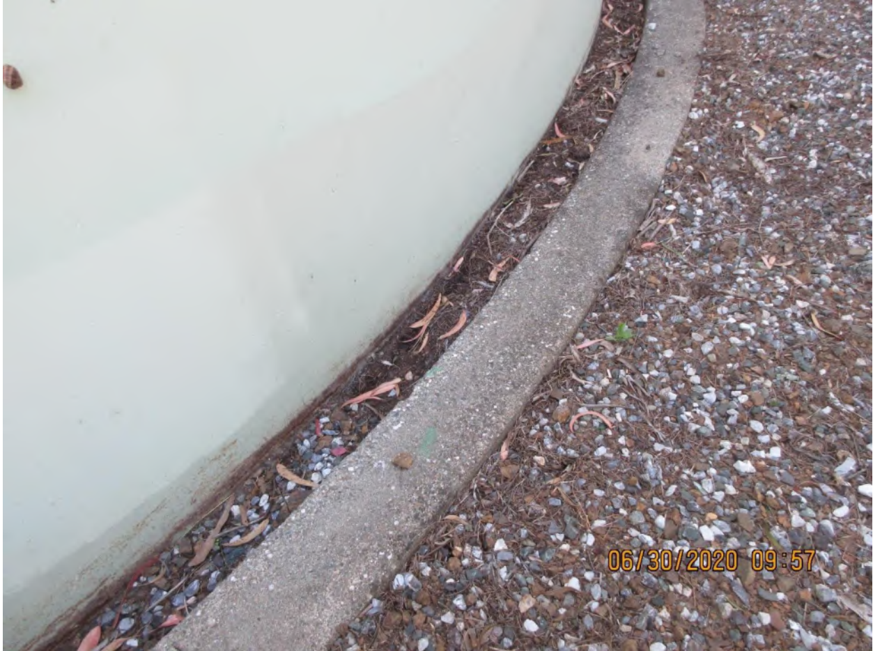
Photo 9: Tank 9 & 10 - Retaining Concrete Ring
