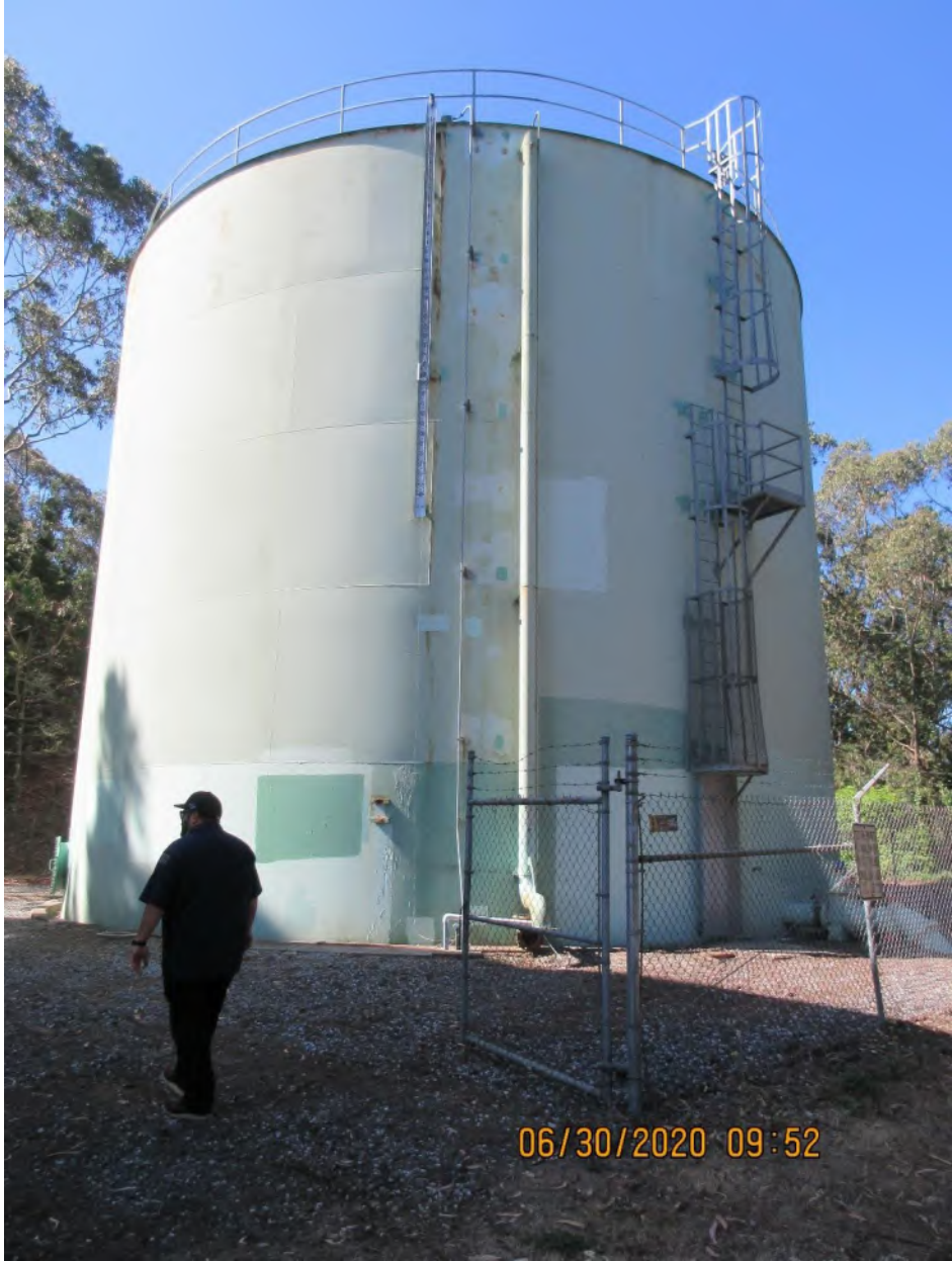
Photo 13: Typical Access Ladder and Roof Railing
