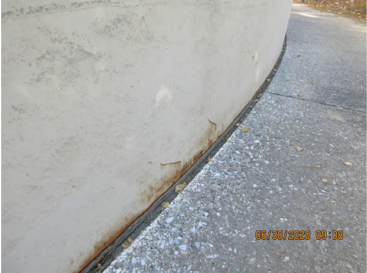
Photo 2: Tank 4 - Concrete Walkway
