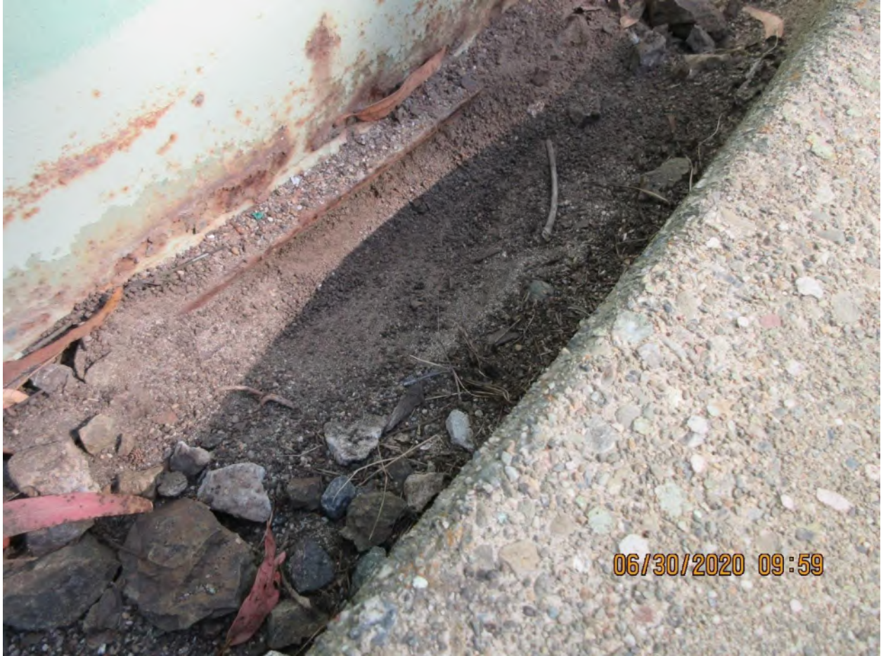
Photo 8: Tanks 9 & 10 - Soil Beneath Bottom Shell of Tank
