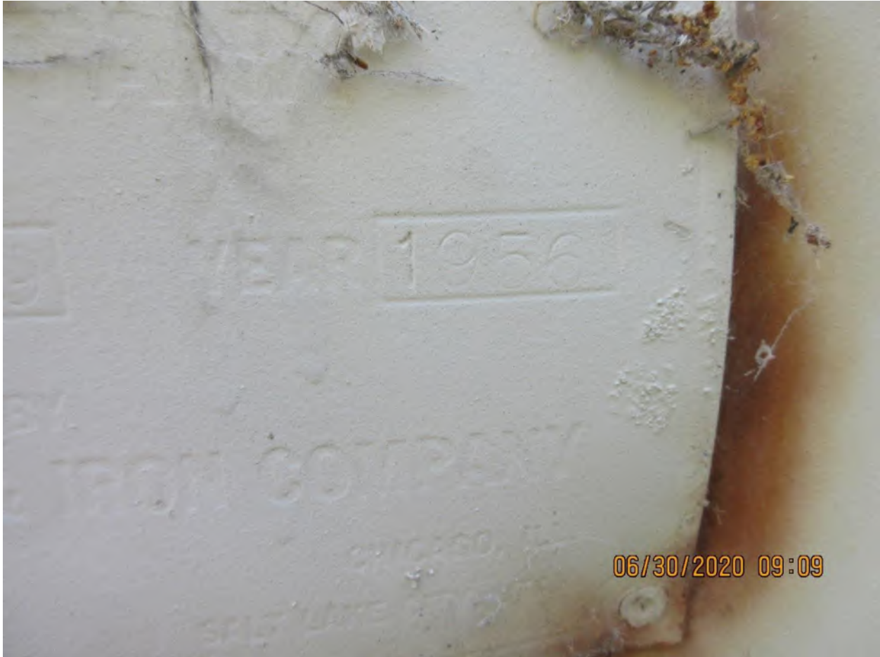
Photo 1: Tank 4 - Year Built
