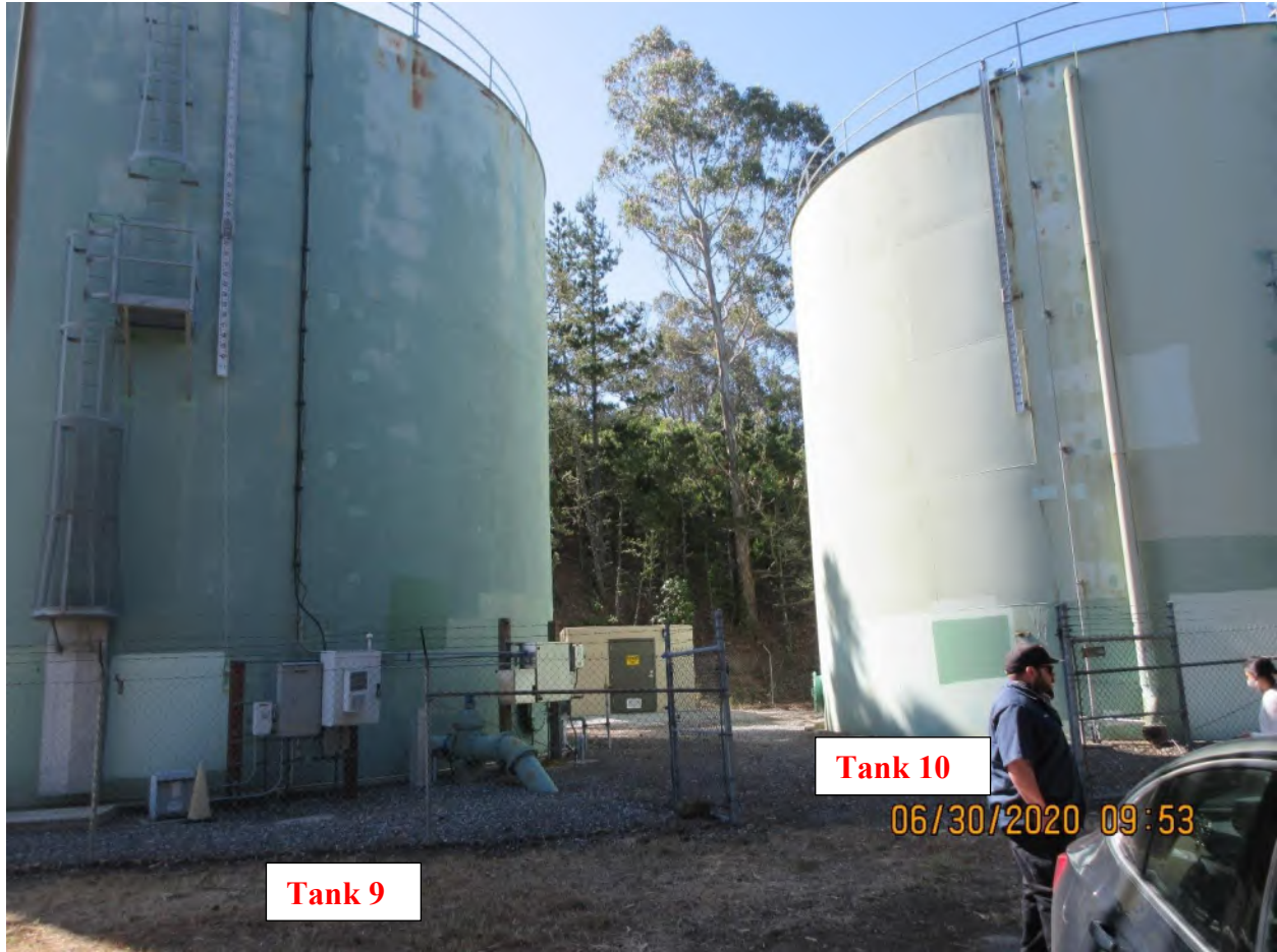
Photo 5: Overview of Tank 9 & 10
