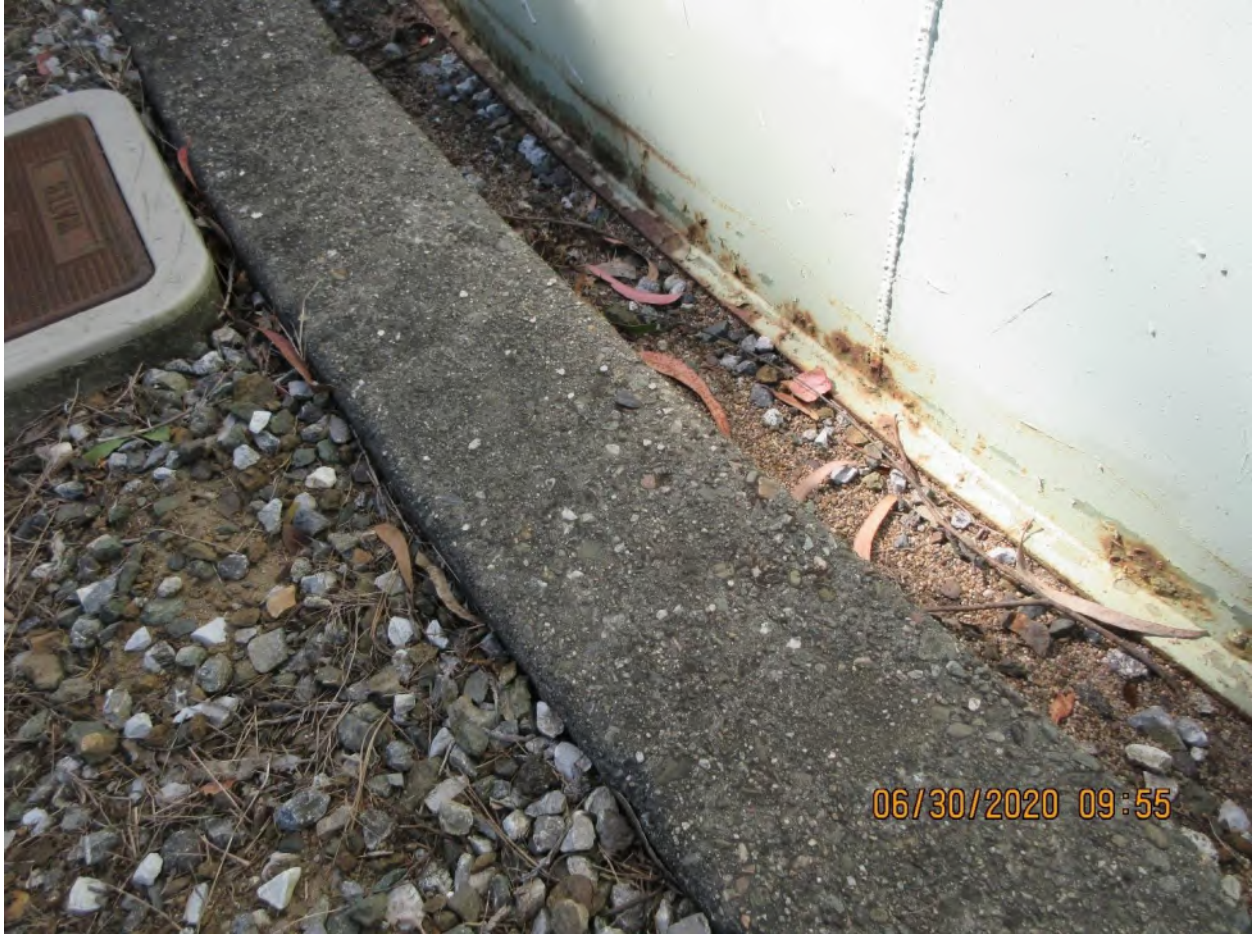
Photo 10: Tanks 9 & 10 - Retaining Concrete Ring
