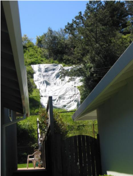
Residential neighborhoods in the city's western hills (top) feature steep topography, some of which is susceptible to landsliding (bottom).
