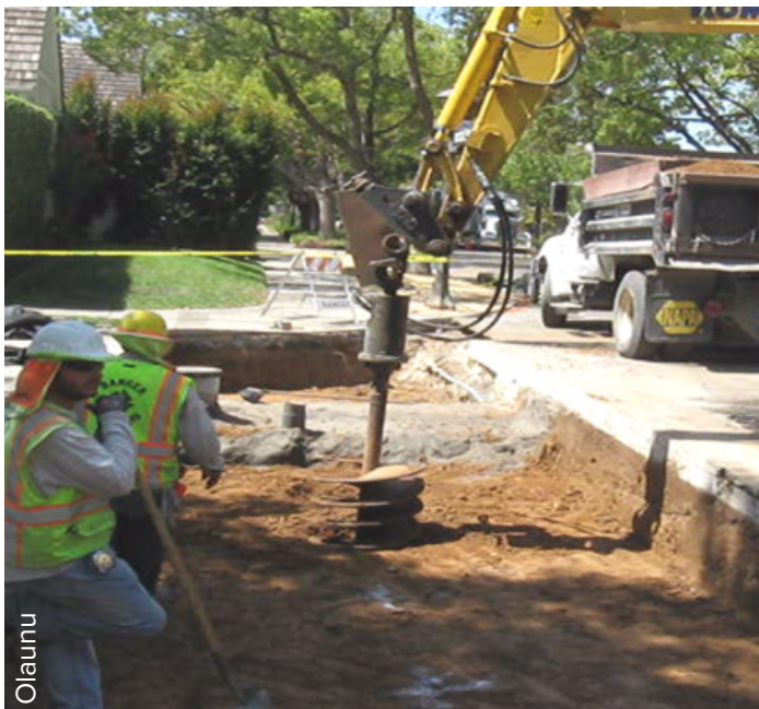
Infiltration Columns Being Constructed on the Peninsula
