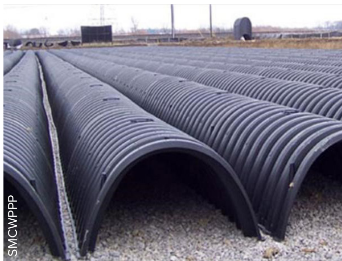
Installation of Subsurface Storage for a Regional Project
